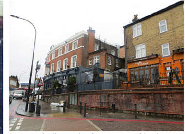
Terrace built on the former canal bed
